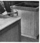
Make counter top of ¾-inch exterior grade plywood, leaving about an inch overhang. Fasten it with aluminum drivescrews, or 2-inch brass screws
