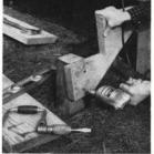
Terrace should be about 8 inches off ground. If ground slopes on approach side, make one step for each 8 inches of rise, using planks 2-by-10 or wider
