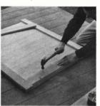
Make simple false-panel doors by nailing 1-by-3s to front and back of thin plywood cut to size of opening. Trim to final size with plane
